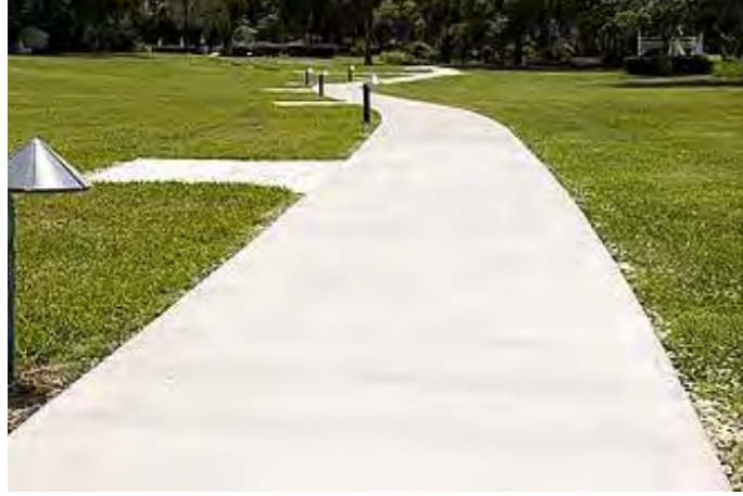
Insitu concrete path
