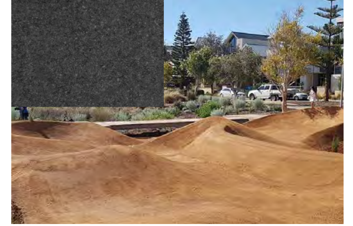
Pump track: Stabilised compacted soil and asphalt top surface
