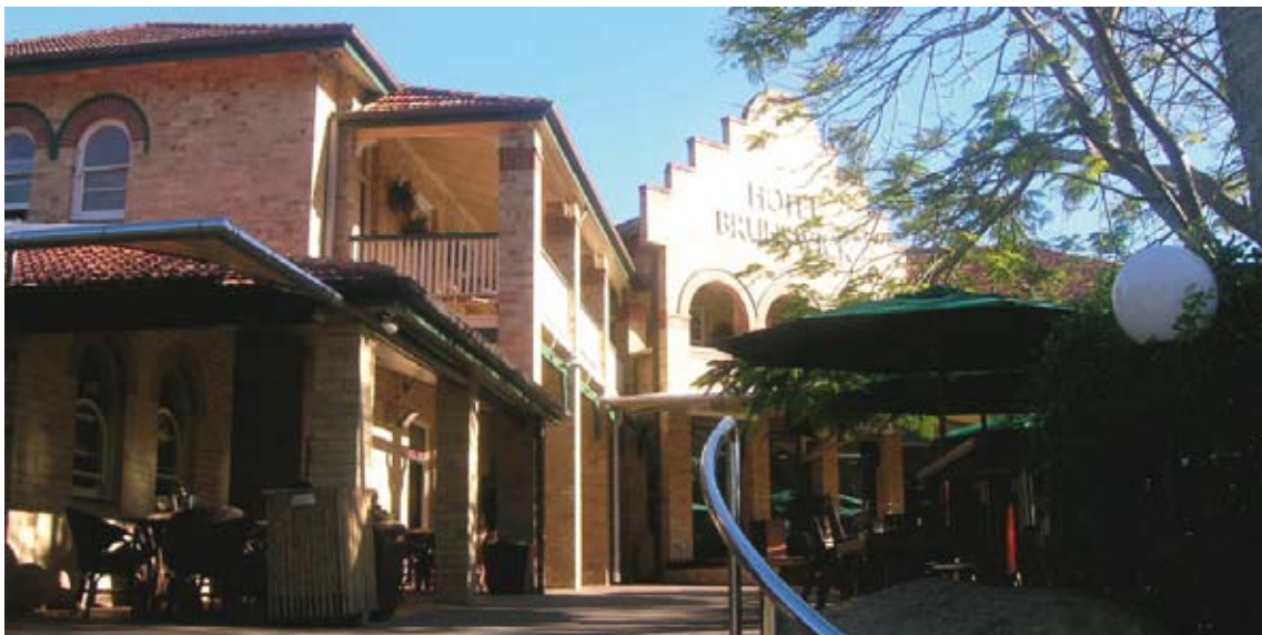
This distinctive public building provides a landmark within the village
