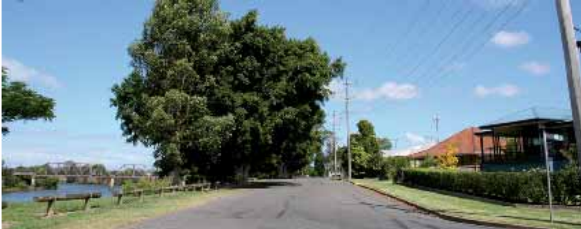
Asymmetric street separating river from residential development; formed kerb and gutter with well maintained grass verge on one side, and grassed swale to the other
