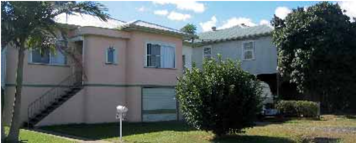
Traditional lightweight elevated housing with garage underneath
