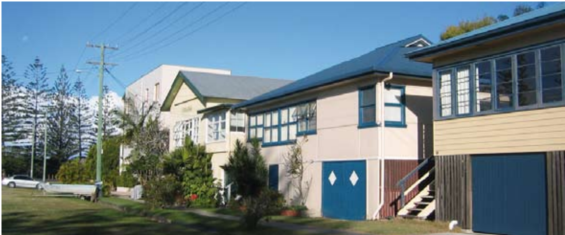
Traditional elevated double level fibro 'flats' built to a consistent setback and building height with internal verandahs and under-croft parking
