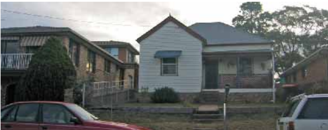
Traditional residential dwelling, elevated and of mixed masonry and lightweight construction with an external verandah
