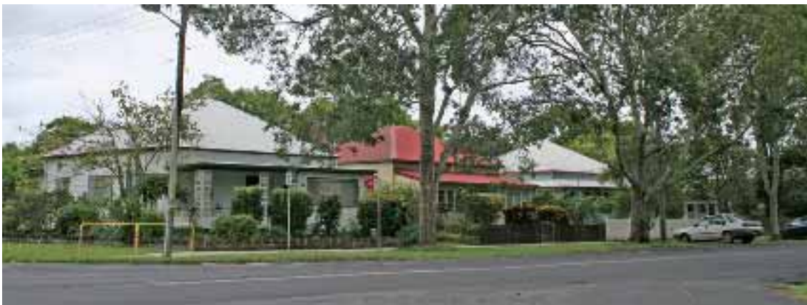
Traditional dwellings with consistent setbacks to front and side boundaries, each with a simple form, built of lightweight materials, elevated slightly above the ground and incorporating a front verandah; all contributing to the character of the town
