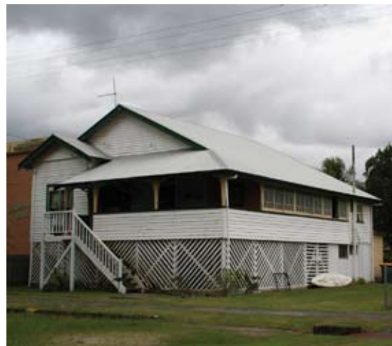
Lightweight, elevated dwelling with strong simple roof form and generous verandah
