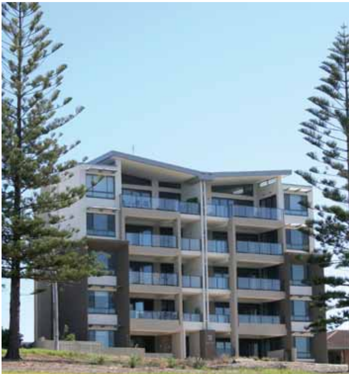
Five storey residential development with strong, component based composition featuring street-side balconies and single service core
