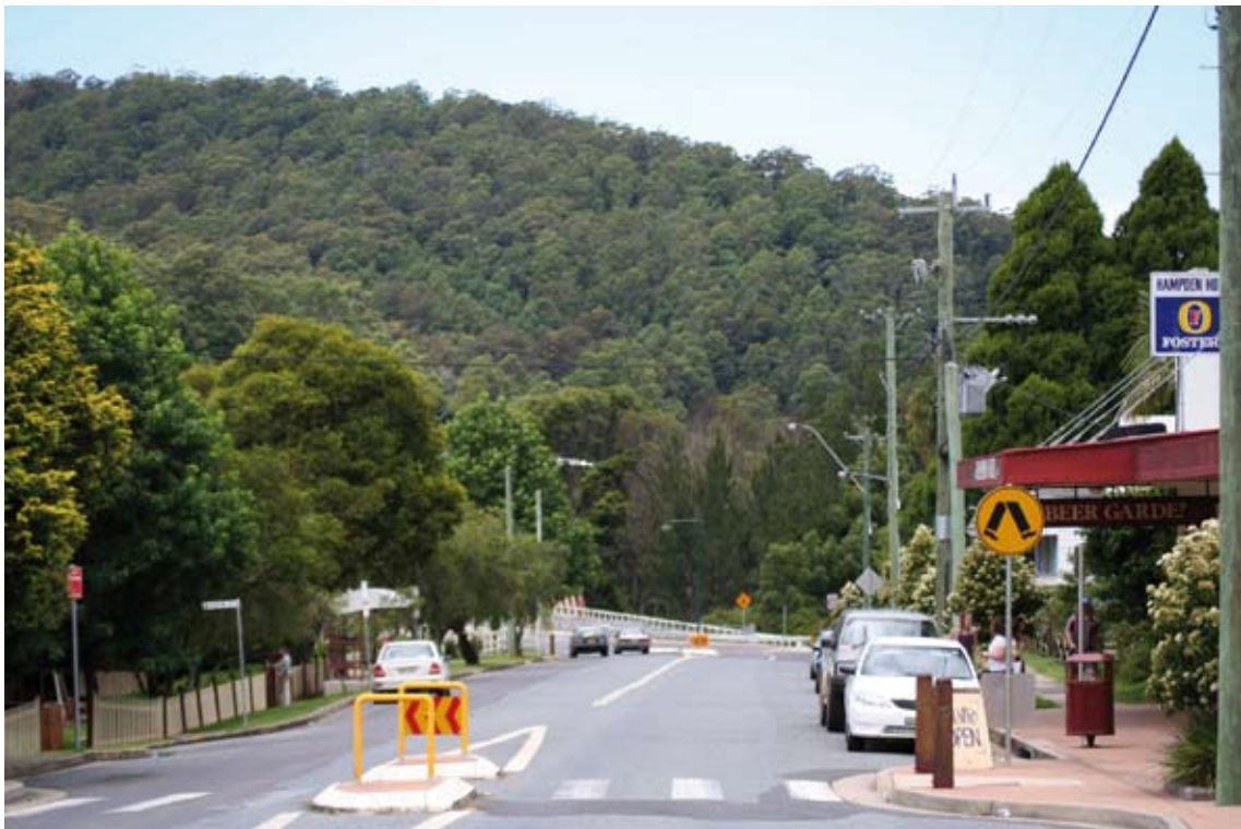
The main street alignment reveals views to the surrounding mountains and includes formed kerb and gutters with footpaths to support commercial uses
