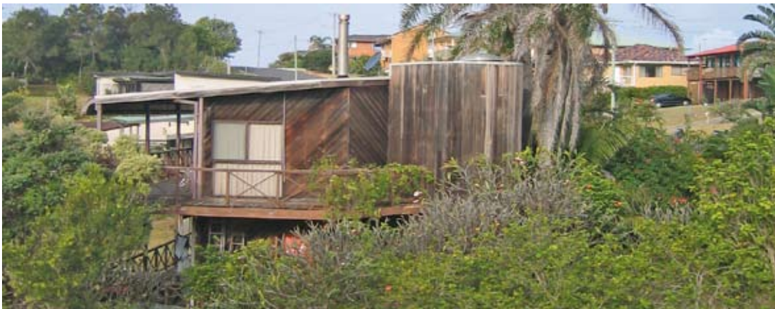
Elevated lightweight dwelling responding to the topography of the village and maximising views to the ocean
