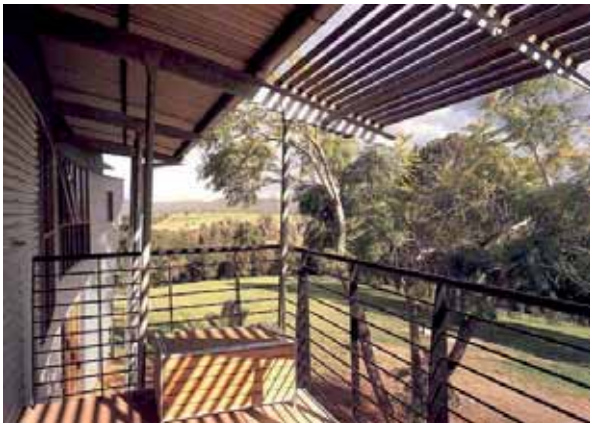
Large eaves and louvred screens shade outdoor living spaces and walls of house, reducing solar gain
