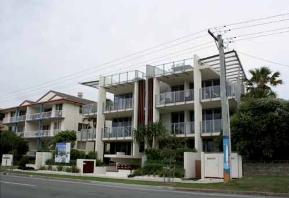
This three storey development with set back and sheltered balconies, echoes the existing rhythms of the streetscape rather than imitating existing built form
