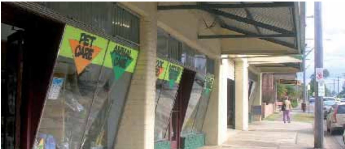
Various building styles characterise the town centre; awnings extending to kerb provide a covered pedestrian path along shop fronts
