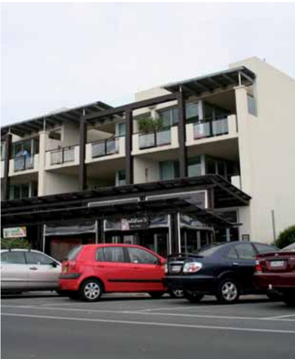
A three storey, mixed development with cafes and retail on the ground floor, residential above; contrasting materials break up the façade, reducing the impact of the volume on the streetscape; easy access to roadside parking is provided
