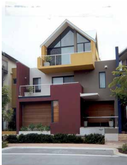
Modern masonry construction; fragmented composition reduces impact of scale on streetscape
