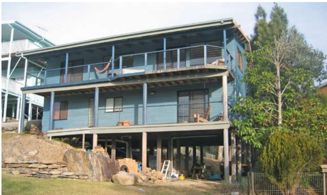
This elevated, lightweight two level dwelling is responsive to the coastal environment maximising views, cross ventilation and passive solar design principals
