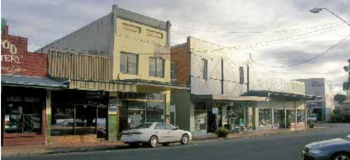
Commercial buildings in town centre typically have a narrow shop front, with awning to the kerb, and utilise parapet forms of consistent alignment
