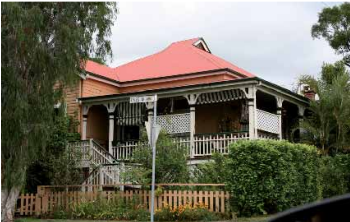
Traditional elevated dwelling of lightweight materials and simple roof form; the verandah is an important extension of internal living space
