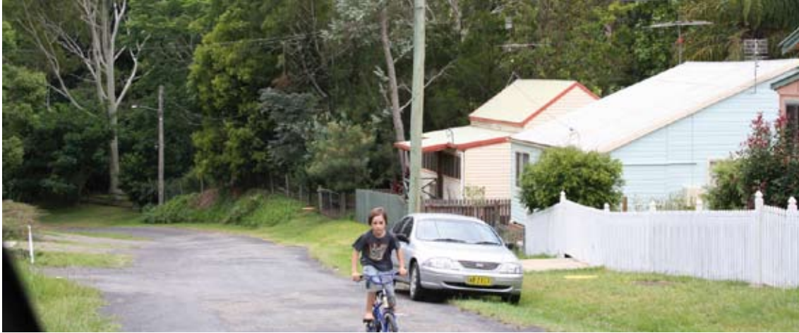
A residential street with narrow unformed carriageway and grassed swales; the river at the bottom of the street gives a strong natural focus to the settlement
