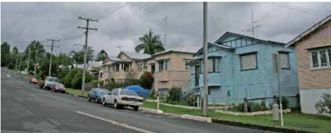
Traditional dwellings of lightweight materials, elevated with internal verandahs and parking; the buildings are aligned consistently along the street
