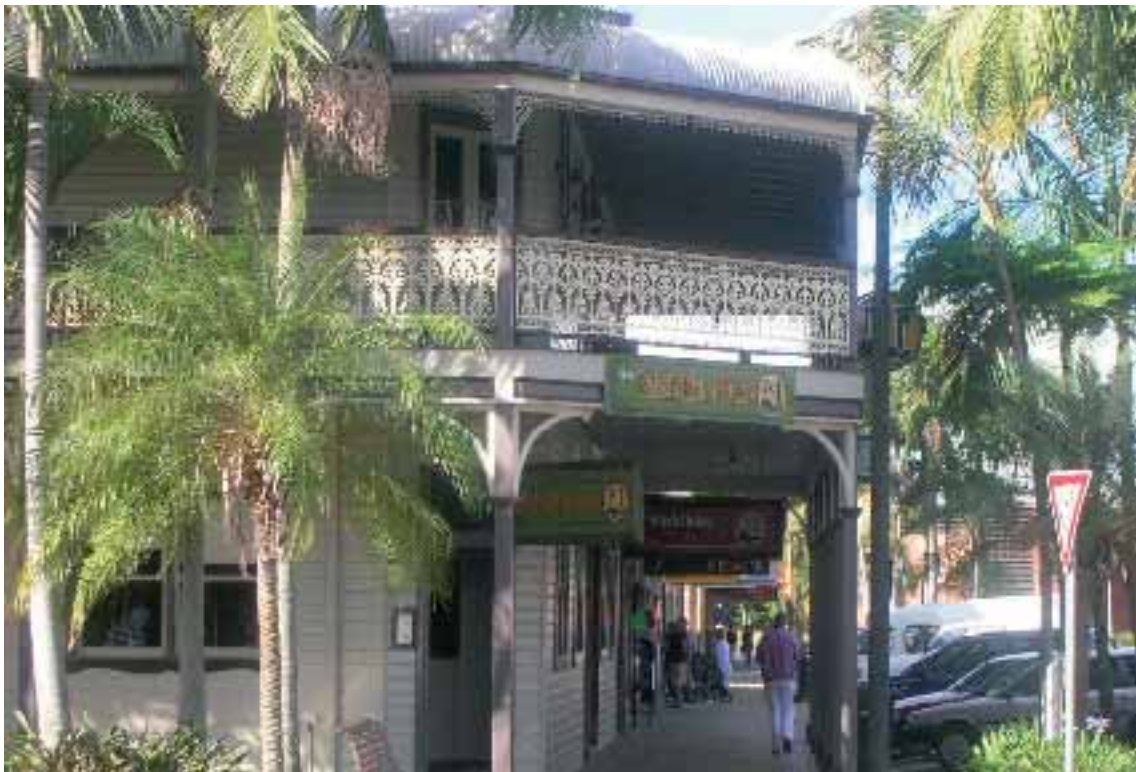
Two storey lightweight commercial building with verandah over footpath, providing a covered pedestrian way
