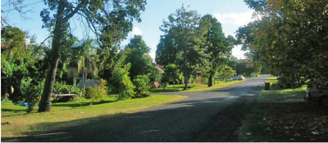
Generous informal road reserve with a relatively narrow carriageway and grassed verges with mature planting
