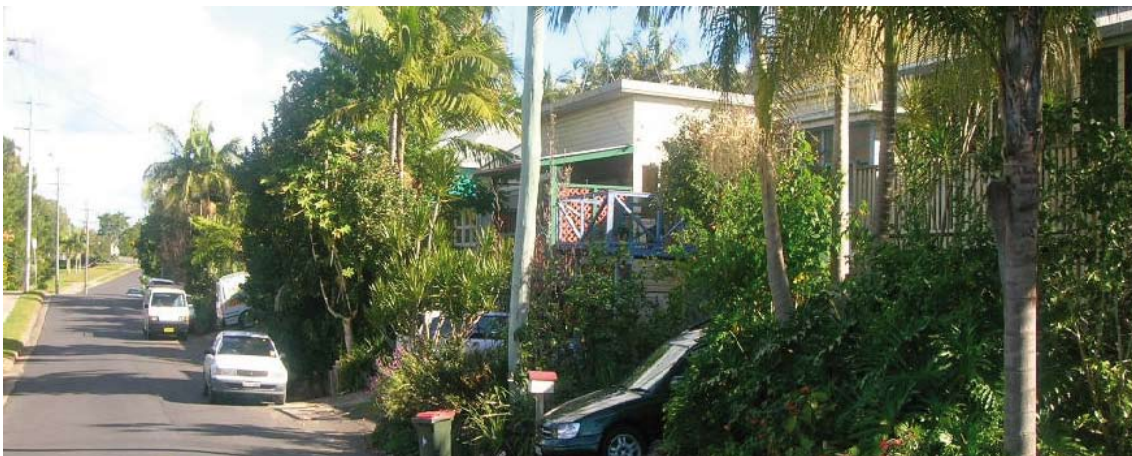
Residential street with informal character, formed kerb and footpath with grassed verge to the lower side of the road; two way carriageway with parking and unformed kerb treatment to the higher side of the road
