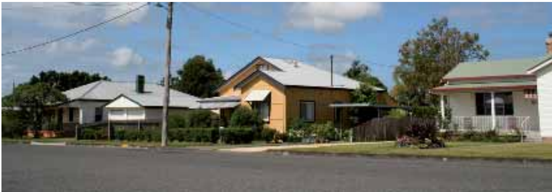
Traditional housing is typically elevated, single level, lightweight, modest detached dwellings with simple roof forms, a consistent alignment to the street and a front porch or verandah
