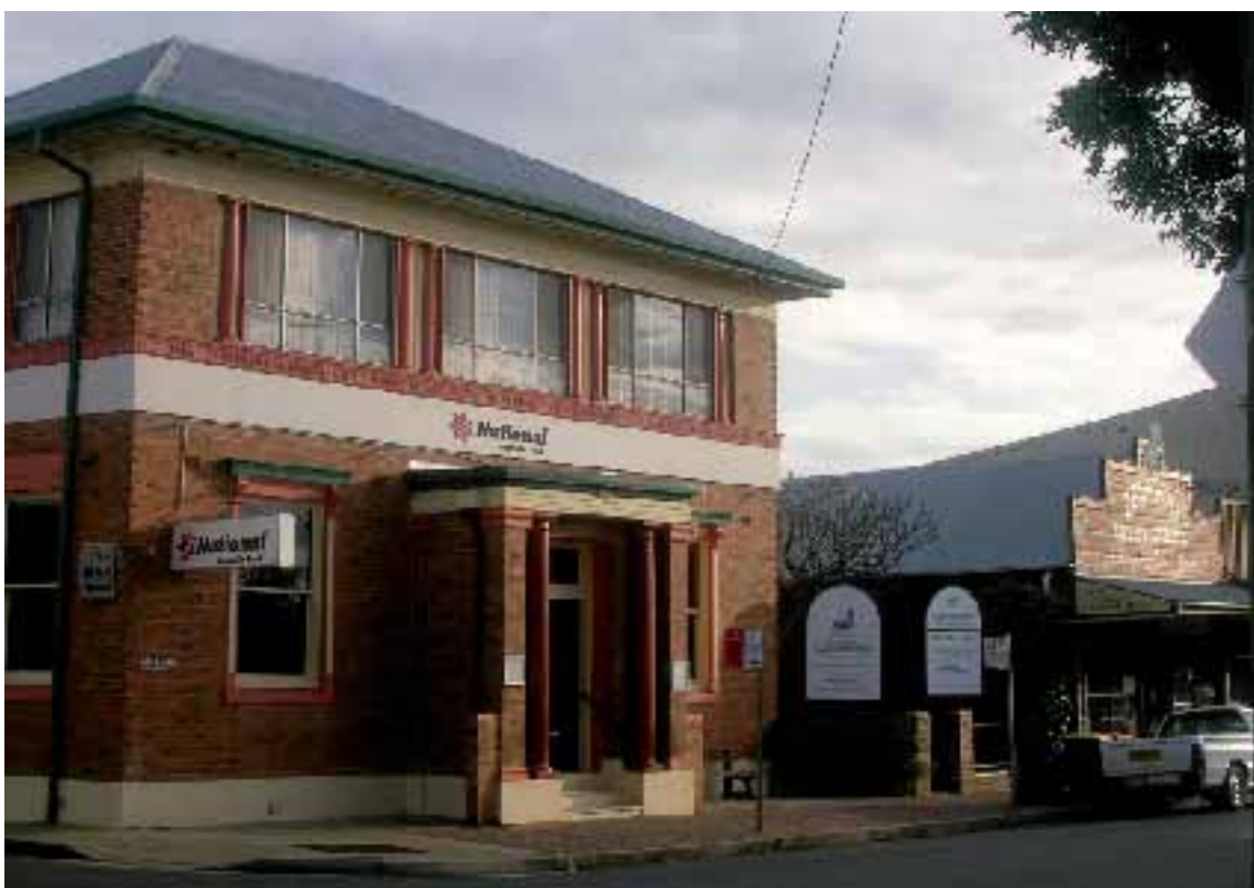
High quality masonry two storey commercial building with a positive address to the street
