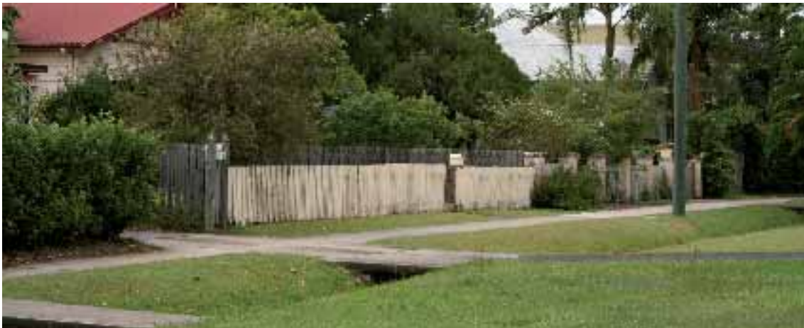
Generous grassed verges with swale drains and defined crossings for vehicles and pedestrian footpaths contribute to a strong streetscape character
