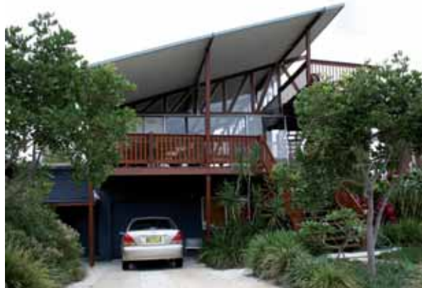
Raised, lightweight structure allows for undercroft parking; clerestory allows sunlight from the east and view to the coast
