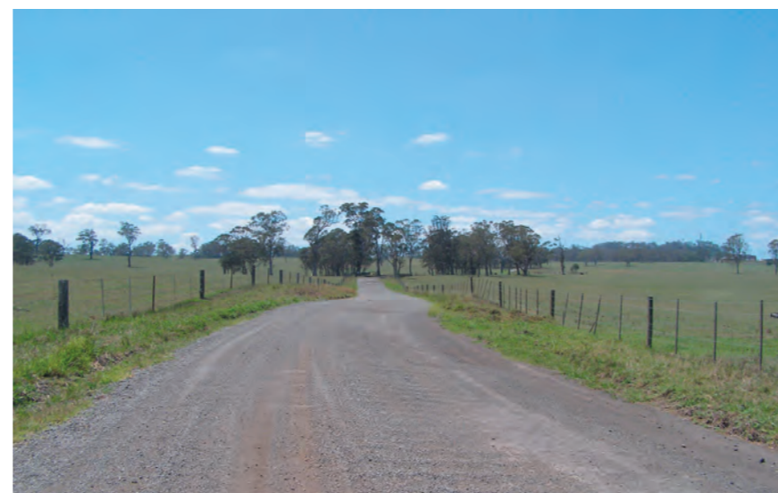
Figure 5 – The existing Badgally Road
