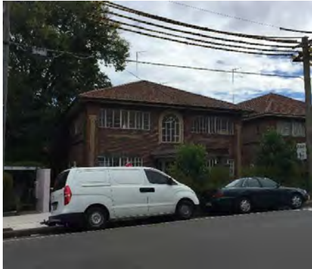
Figure 4 – Façade of 66 Ewart Street, Dulwich Hill.
