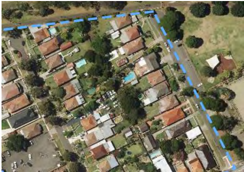
Figure 26 - Excerpt from Figure 68 of the initial Heritage Review report showing an aerial view of the Group A sites.
