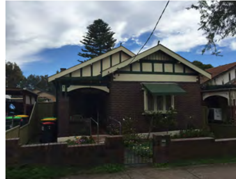
Figure 18 — Detail of a dwelling within Group A
