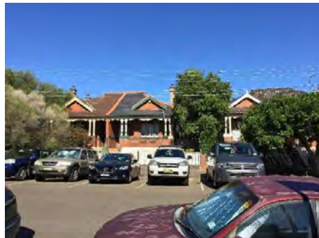
Figure 13 - View of 6-8 Warburton Street, Marrickville
