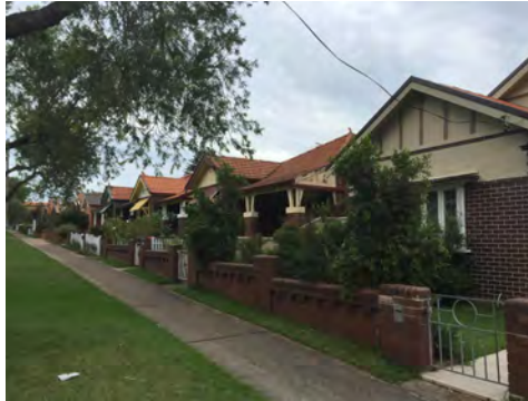
Figure 17 — Looking north along Cleary Street at the Group A buildings
