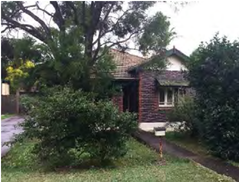
Figure 28 – Pre WW1 dwelling in Acacia Street
