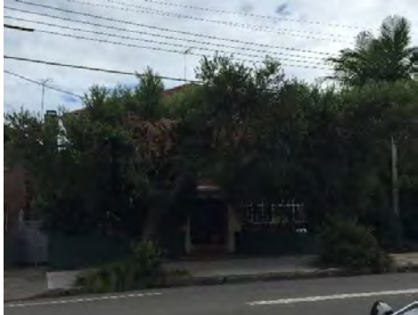
Figure 5 - Façade of 68 Ewart Street, Dulwich Hill.
