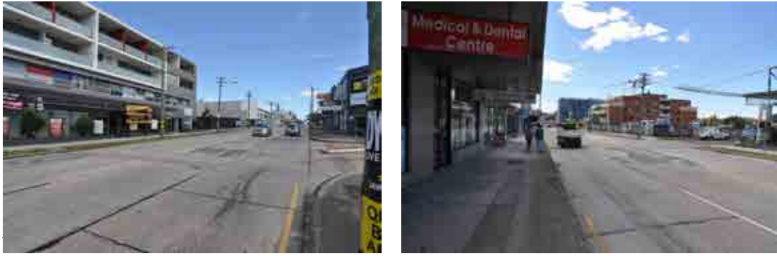
Canterbury Road - depressed retail environment
