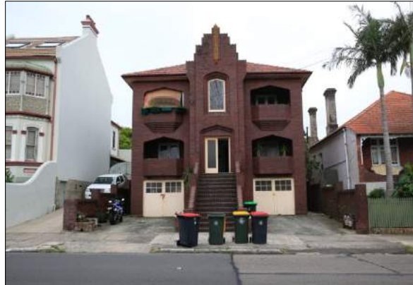
Figure 2: Looking at the front elevation of the subject site.
