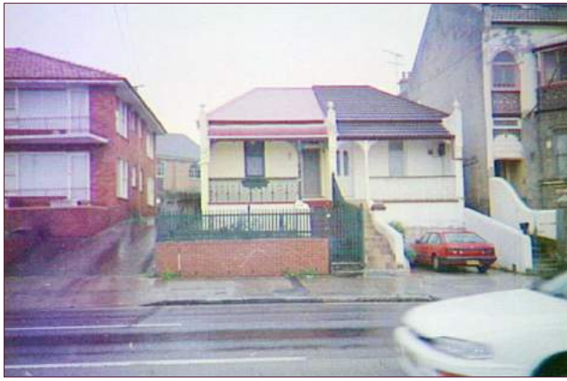
Figure 3: No. 39-41 Canterbury Road, Hurlstone Park 1998.
