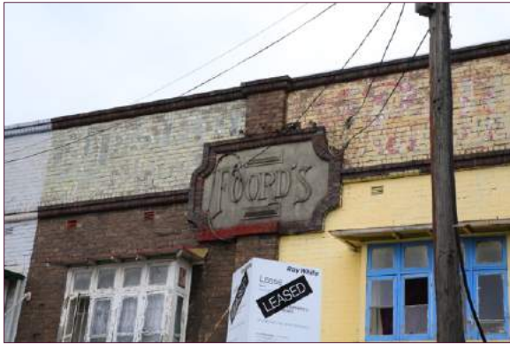
Figure 1: "Foord's" plaque on the building parapet.
