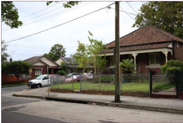
Figure 1: Looking at the front elevation of the subject site.
