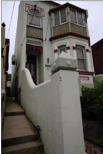
Figure 1: Looking at the front elevation of the subject site.
