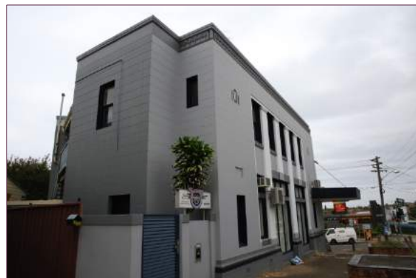
Figure 2: Looking at the rear elevation of the subject site.
