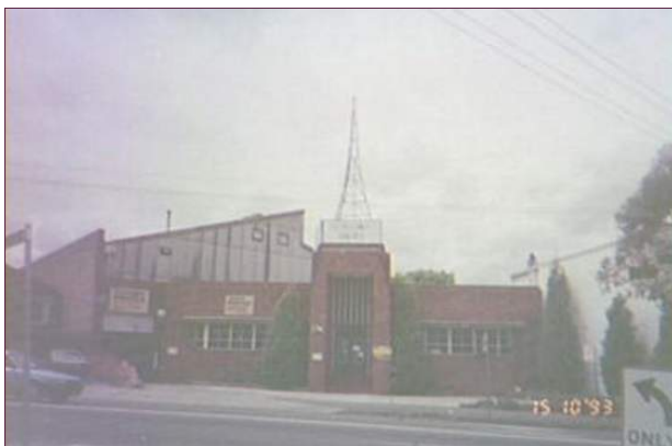
Figure 3: No. 174 Canterbury Road, Canterbury, 1993. Evidence of face brick prior to rendering of the façade.
