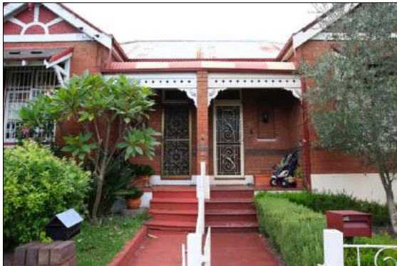
Figure 1: Looking at the front steps and entrance of the subject site.
