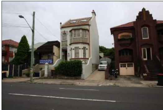
Figure 4: Looking at the front elevation of the subject site.
