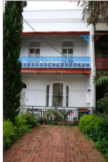
Figure 4: Looking at the front elevation of No. 68 Canterbury Road, Canterbury.
