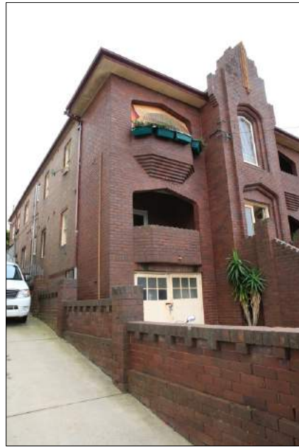
Figure 4: Looking toward the front elevation of the subject site.
