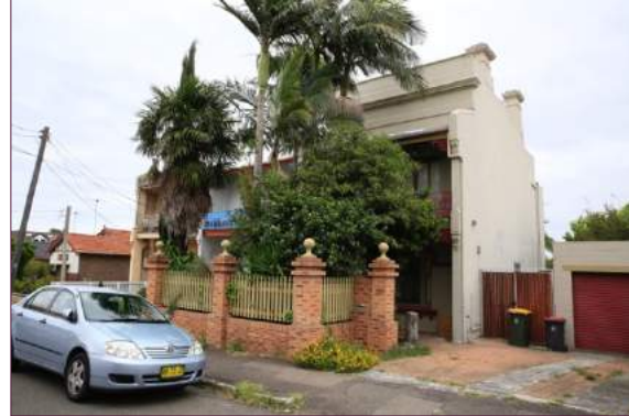
Figure 2: Looking at front elevation of No. 70 Minter Street.
