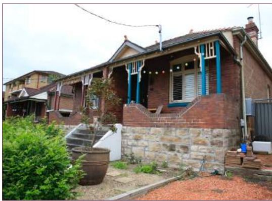
Figure 3: North-easterly view of the front façade of No. 19 & 21 Jeffrey Street.
