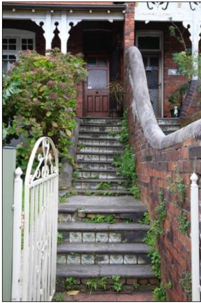
Figure 3: Looking at the front steps and front entrance of No. 31 Canterbury Road, Canterbury.
