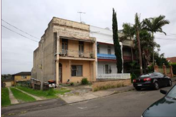
Figure 1: Looking at terrace row from Minter Street.
