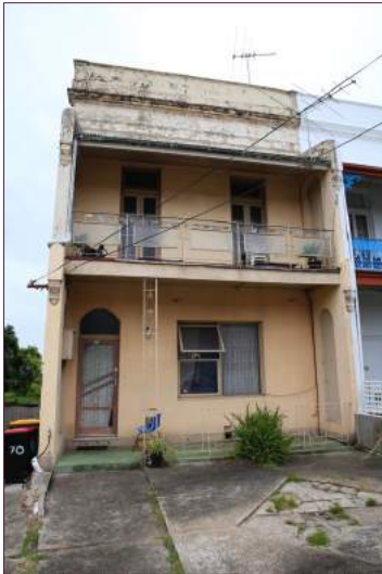
Figure 3: Looking at the front elevation of No. 66 Canterbury Road, Canterbury.
