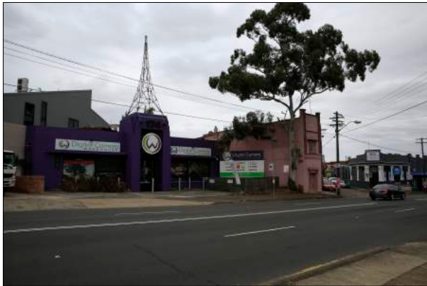
Figure 1: Looking south east along Canterbury Road.
