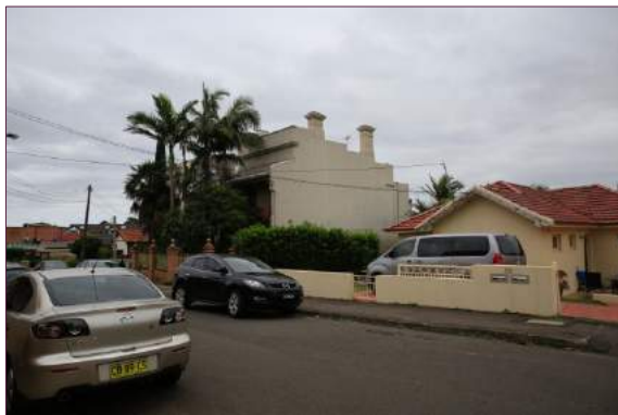
Figure 4: Looking opposite from the subject site toward the western side of Minter Street.
