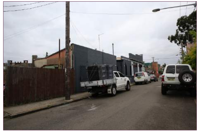
Figure 2: Looking toward the rear and side elevation of the subject site from Minter Street.
