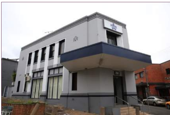
Figure 1: Looking at the side elevation of the subject site.
