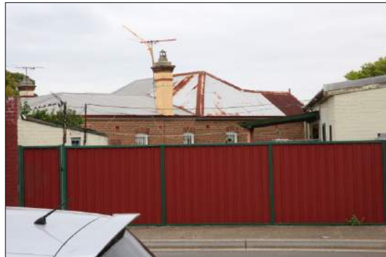
Figure 2: Looking at the side elevation of the subject site.
