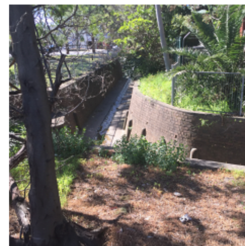
7. Salt Pan Creek stormwater channel
