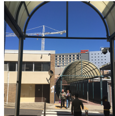
Covered arcades link the station with the Sports Centre
