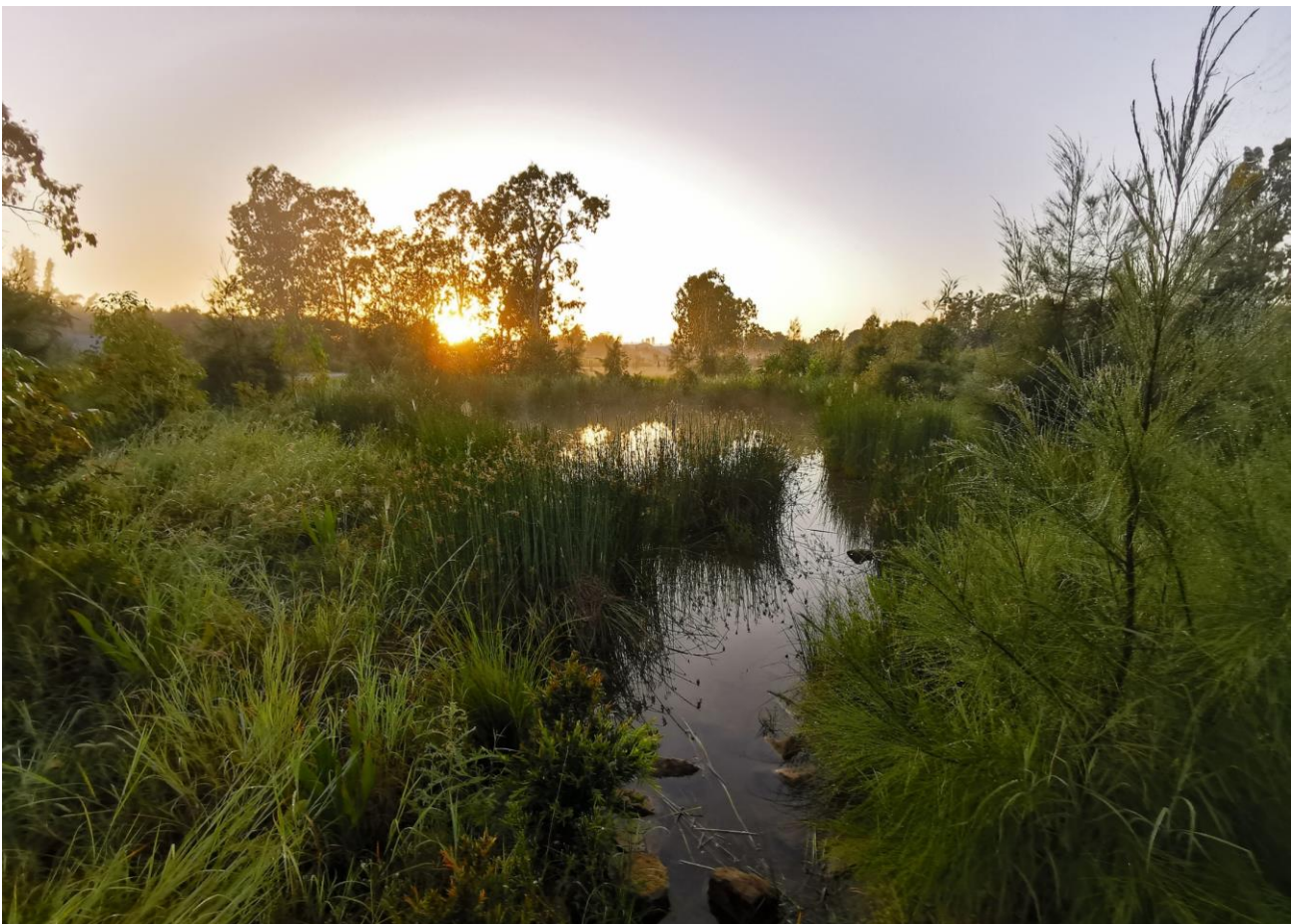
Figure 14: Example of stormwater infrastructure
