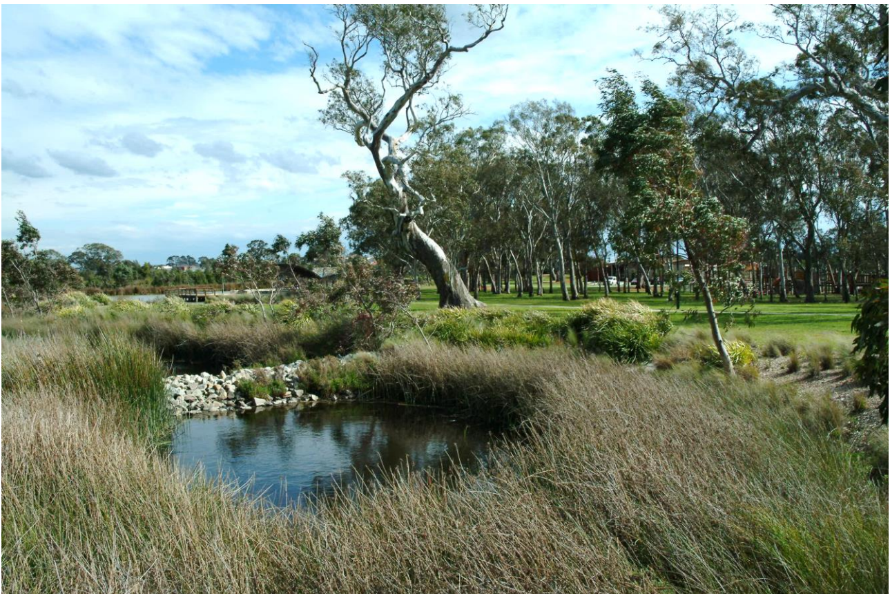
Figure 13: Example of stormwater assets serving multiple uses
