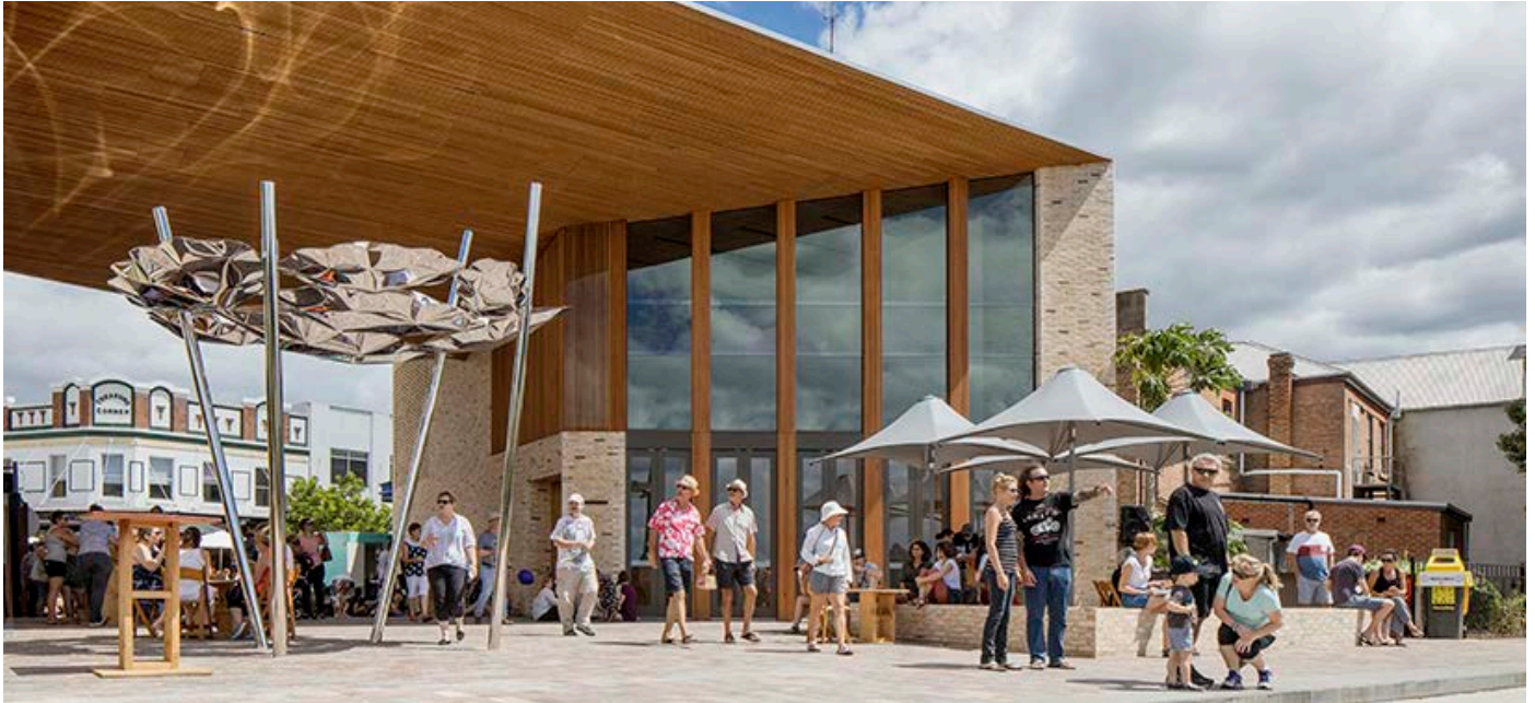
Figure 82 - Extending the main street to the river, supporting a revitalisation of the central business precinct - Maitland Riverlink, Maitland.
