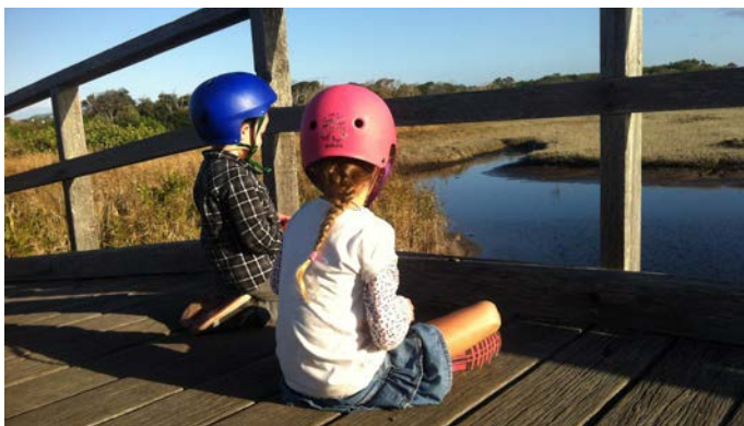
Figure 79 - Creek bridges connect the Suffolk community through the Tallow Creek Wetland Area to a number of key amenities such as schools, shops the beach - Tallow Creek Pathway, Suffolk Park.
