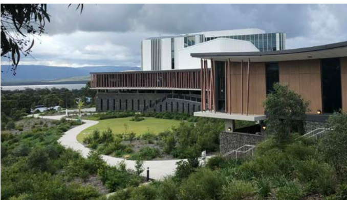
Figure 83 - Landform manipulation of drainage corridor to create an active open space and recreational link - Shellharbour Civic Centre, Shellharbour.
