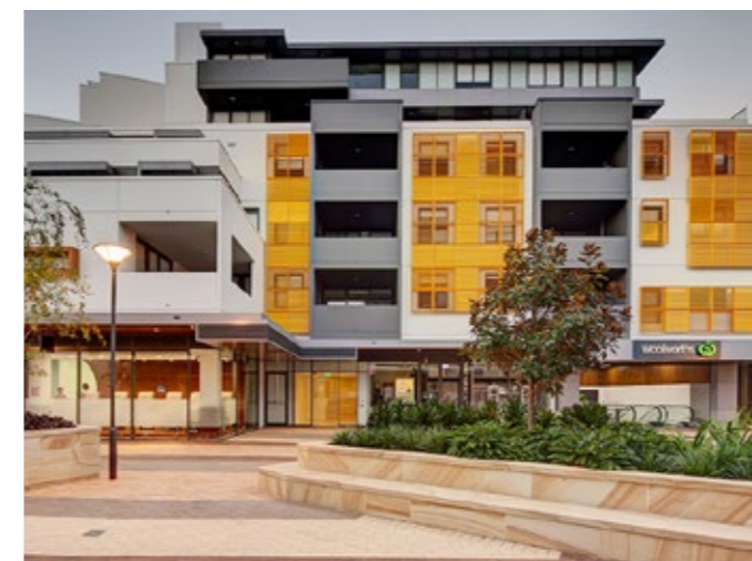
Figure 25: Proposed location of mixed use retail & residential, and desired character and built form
