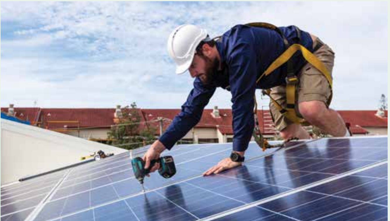
Solar panel technician
