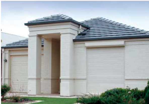
Figure 3.28: Examples of roller shutters over window openings
